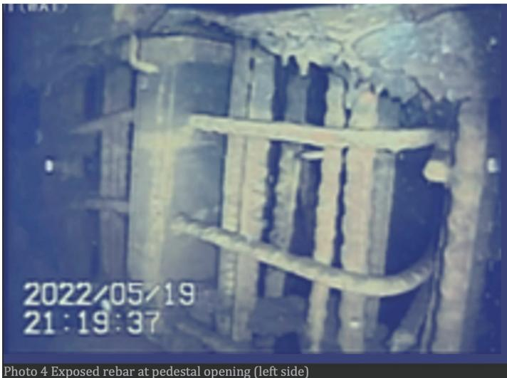
Photo 4 Exposed rebar at pedestal opening (left side)
